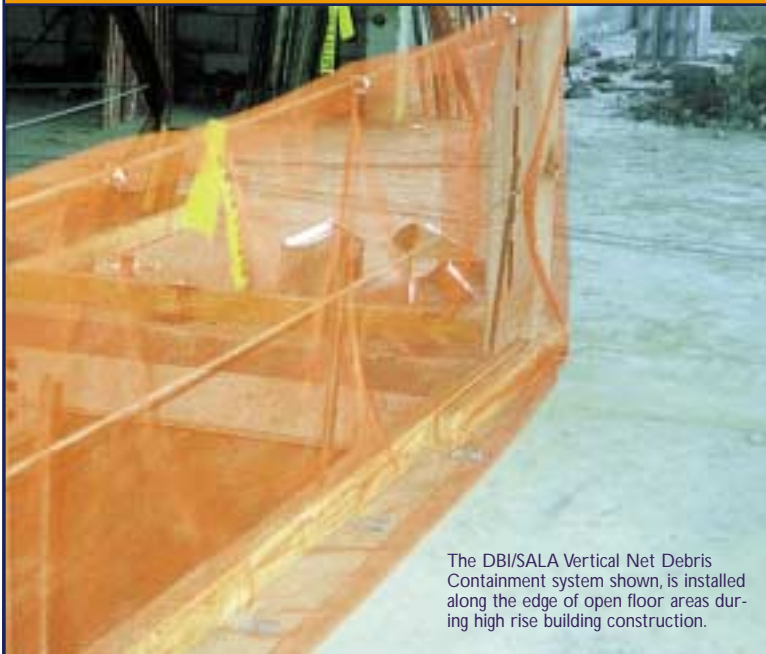
Zip-Clips provide a simple means of installing and removing the net from a standard cable set up.
